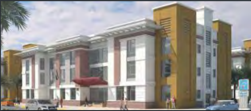
ADNOC Bachelor Accommodation Client: Abu Dhabi National Oil Company for Distribution (14 Buildings) in Abu Dhabi, U.A.E. Contractor: Target
