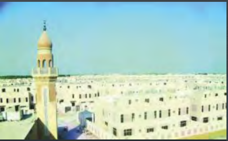
GOSI Residential project , Jubail in Saudi Arabia 400 low rise towers and villas Main Contractor: Azmeel Consultant: Sofcon
