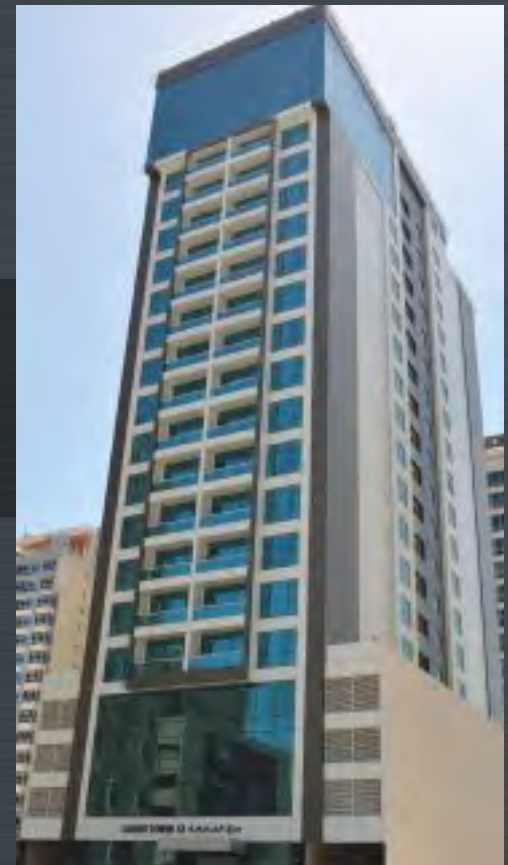
Luxury Tower 1 in Bahrain 20 storey building at Juffair
