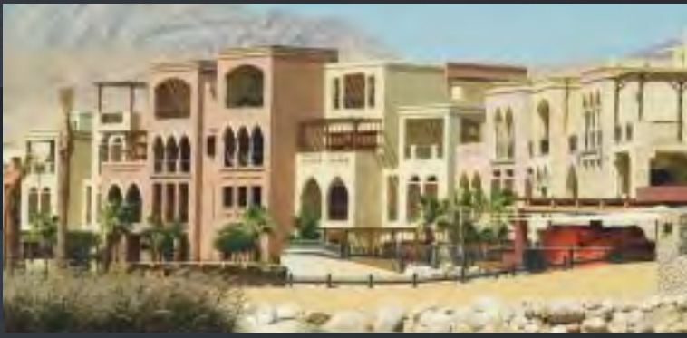
Tala Bay Resort , in Aqaba, Jordan Client: Jordan projects for Tourism Development Consultant: Mohammed Mahmoud Abu Afifa Office Main Contractor: Aqaba Gulf Contracting Company
