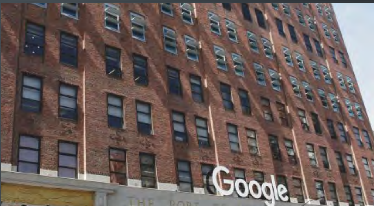
Google 111 8th Ave, NY (Google) New York, USA General Contractor: Taconic Management Comp Architect: HWL International, LLP Ext. Wall Consultant: Gilsanz Murray Stefcsek LLP
