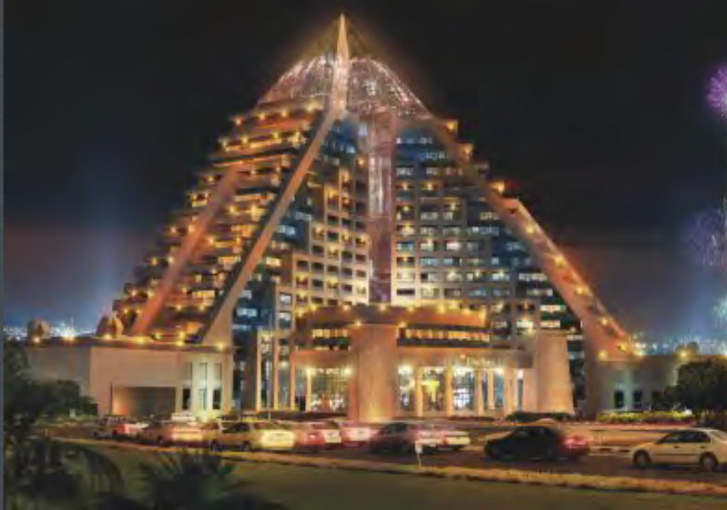
Raffles Hotel & Wafi Mall Phase Extension Client: MKM Commercial Holdings LLC (pyramid shape), Wafi City, Dubai, UAE Main Contractor: Khansaheb Civil Engineering Consultant: Arif & Bintoak
