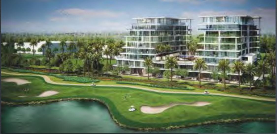
AKOYA G+7 Golf Apartments Client: Damac Crescent Properties LLC Dubai, U.A.E. Consultant: Atkins Main Contractor: Various
