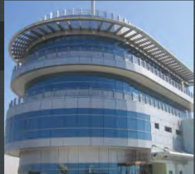
Dubai Maritime City Control Building, Dubai, U.A.E.
